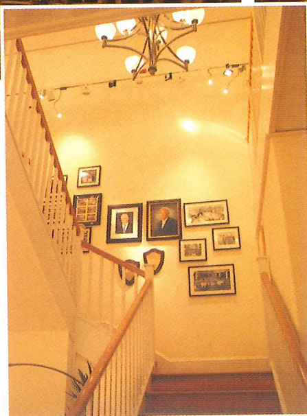
Climbing the stairs to the second floor, customers notice a large foyer fixture (equipped with a chandelier lift system), an array of cable and track lights whose individual beam characteristics are demonstrated on the wall, and the family gallery of photos.
