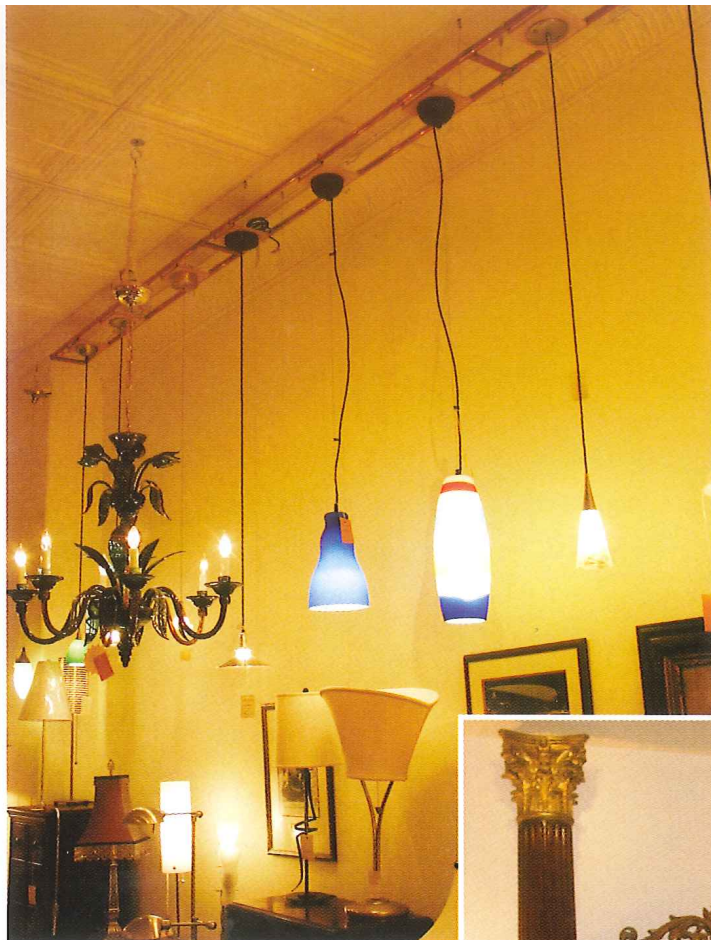
Inspired by a showroom in Boston, Kurland suspended copper tubing to display a row of pendants without destroying the building's original tin ceilings.
